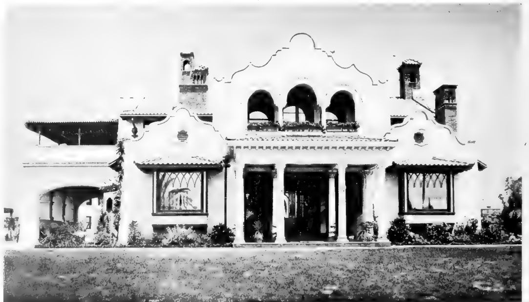
House of Brigadier-General H. G. Otis, Los Angeles, California
